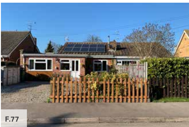
Figure 77: The original building should remain the dominate element of the property. The front extension is not of a sympathetic scale. The flat roof should be avoided in any future developments.
