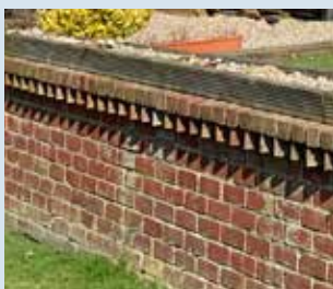
Low wall built with red brick
