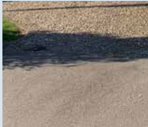
Mix of gravel and paving
