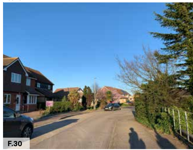
Figure 30: Local example of a permeable road, Drake Avenue, which connects The Drive to Nipsells Chase
