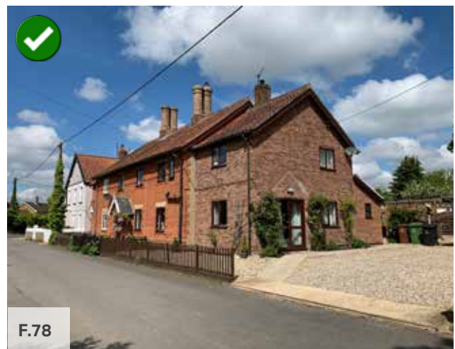
Figure 78: Positive example of side extension which complements the scale of the existing property, somewhere in the UK.
