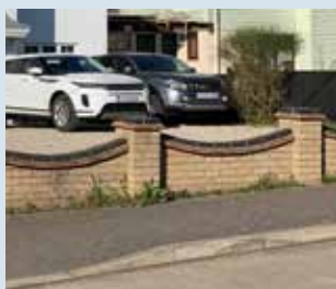
Low wall built with gault brick
