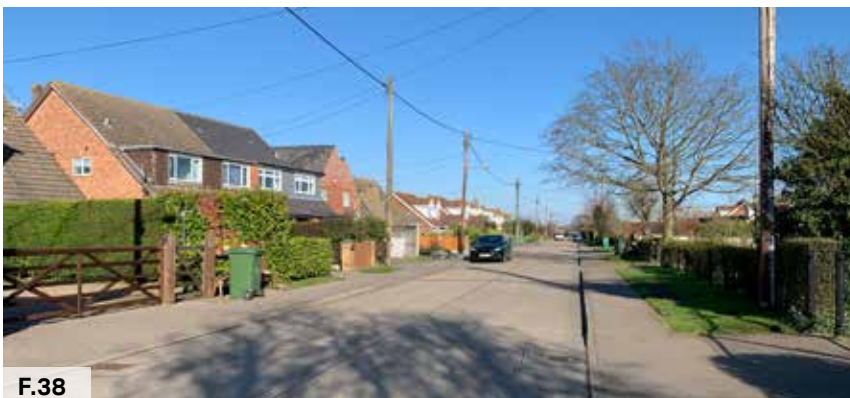
Figure 37: Cross-section to illustrate some guidelines for a Residential Street Type 2. Figure 38: Local example of a Residential Street Type 2, West Avenue.
