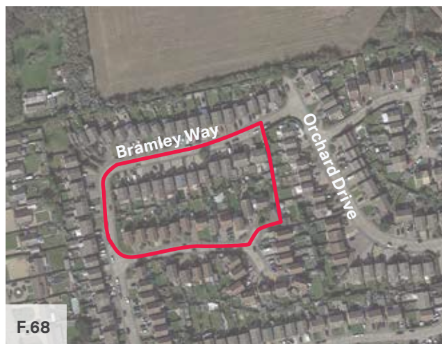
Figure 68: Example of higher density development on Bramley Way with reduced green spaces and gaps between properties.
