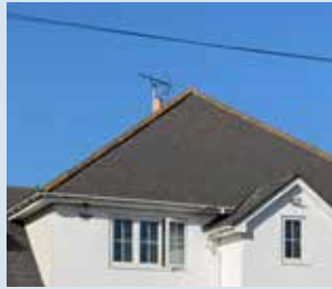
Hipped roof built with slate
