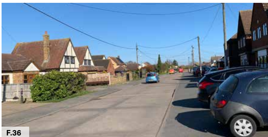
Figure 35: Cross-section to illustrate some guidelines for a Residential Street Type 1. Figure 36: Imperial Avenue as one of the main roads in Mayland.
